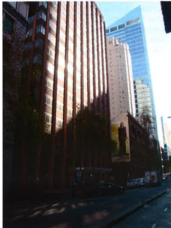
Figure 3: 443-451 Kent Street Sydney as at May 2014
